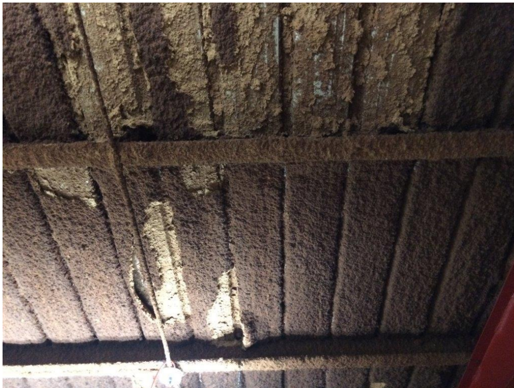
Photo 2: Spray Applied Ceiling Insulation
