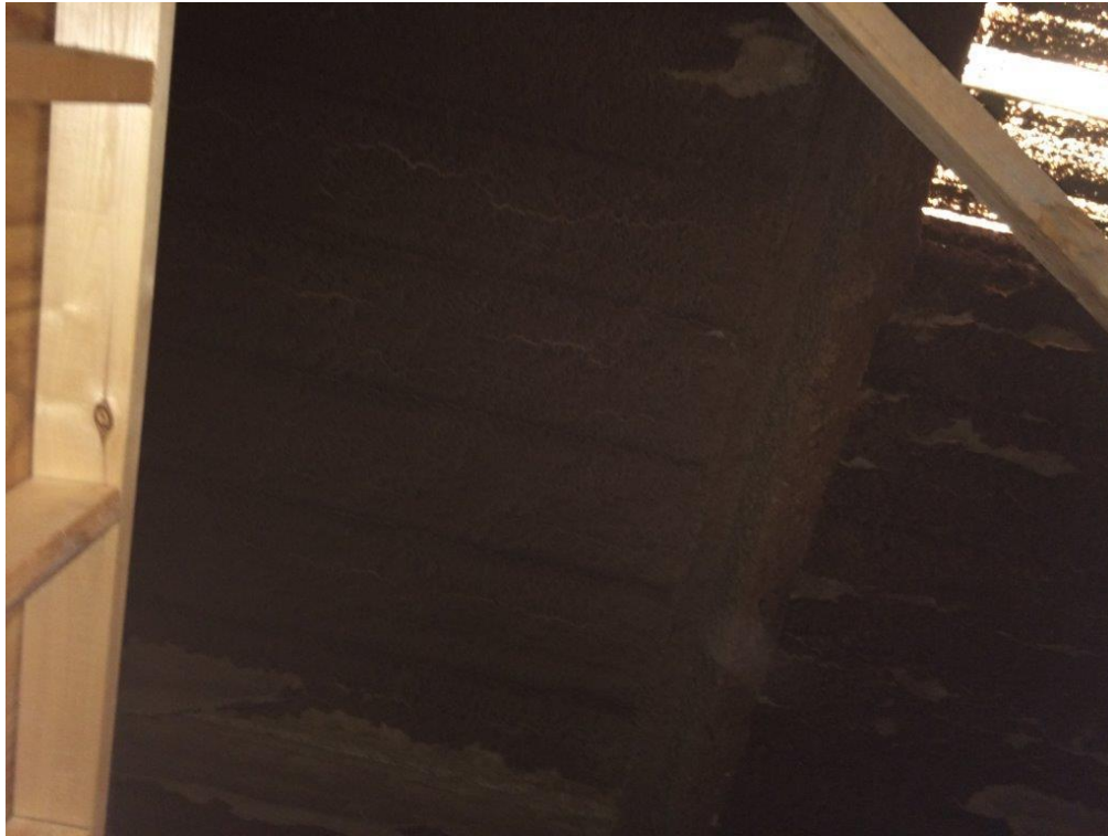
Photo 1: Spray Applied Ceiling Insulation
